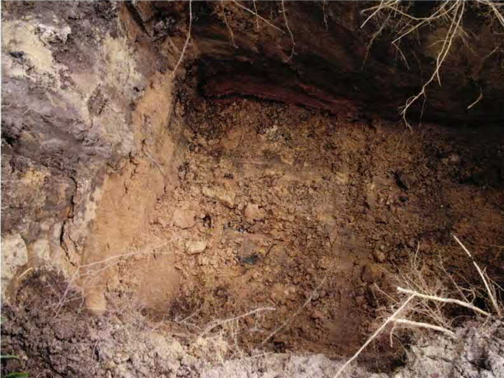
Picture 2: UST 825Azalea excavation in progress.
